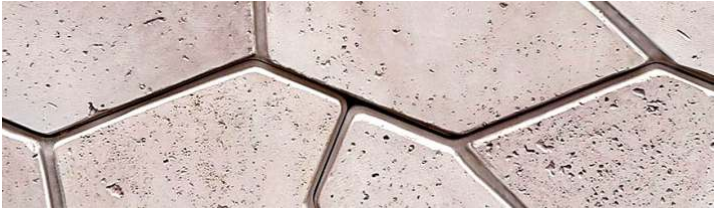
PANEL CONNECTIONS BEFORE GROUTING
