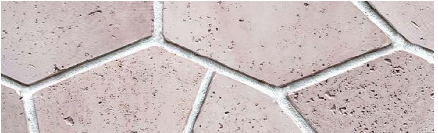
PANEL CONNECTIONS AFTER GROUTING
